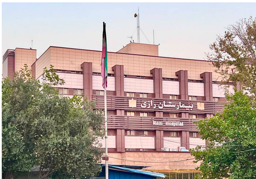
Fig. 1: The hospital view from its new building structure
